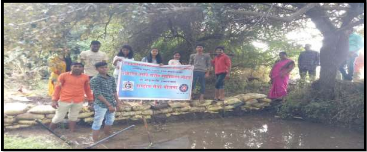
NSS volunteers constructed Vanrai Bandhara at Malegaon during the Camp
