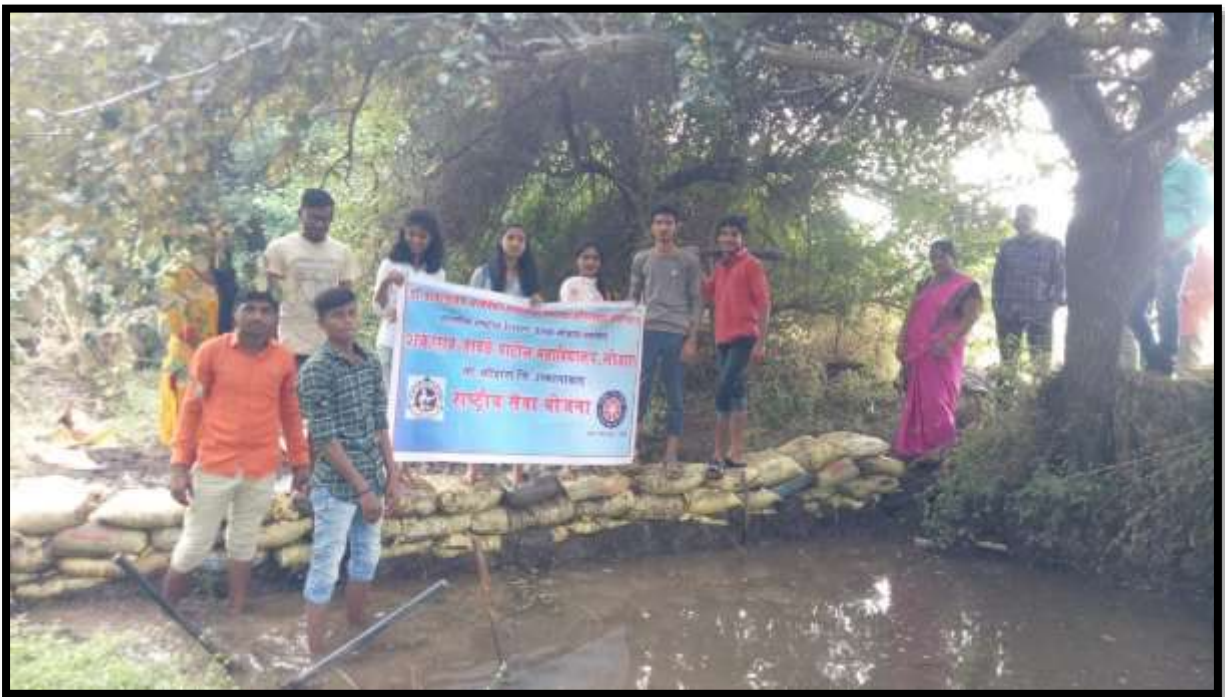
NSS volunteers constructed Vanrai Bandhara at Malegaon during the Camp
